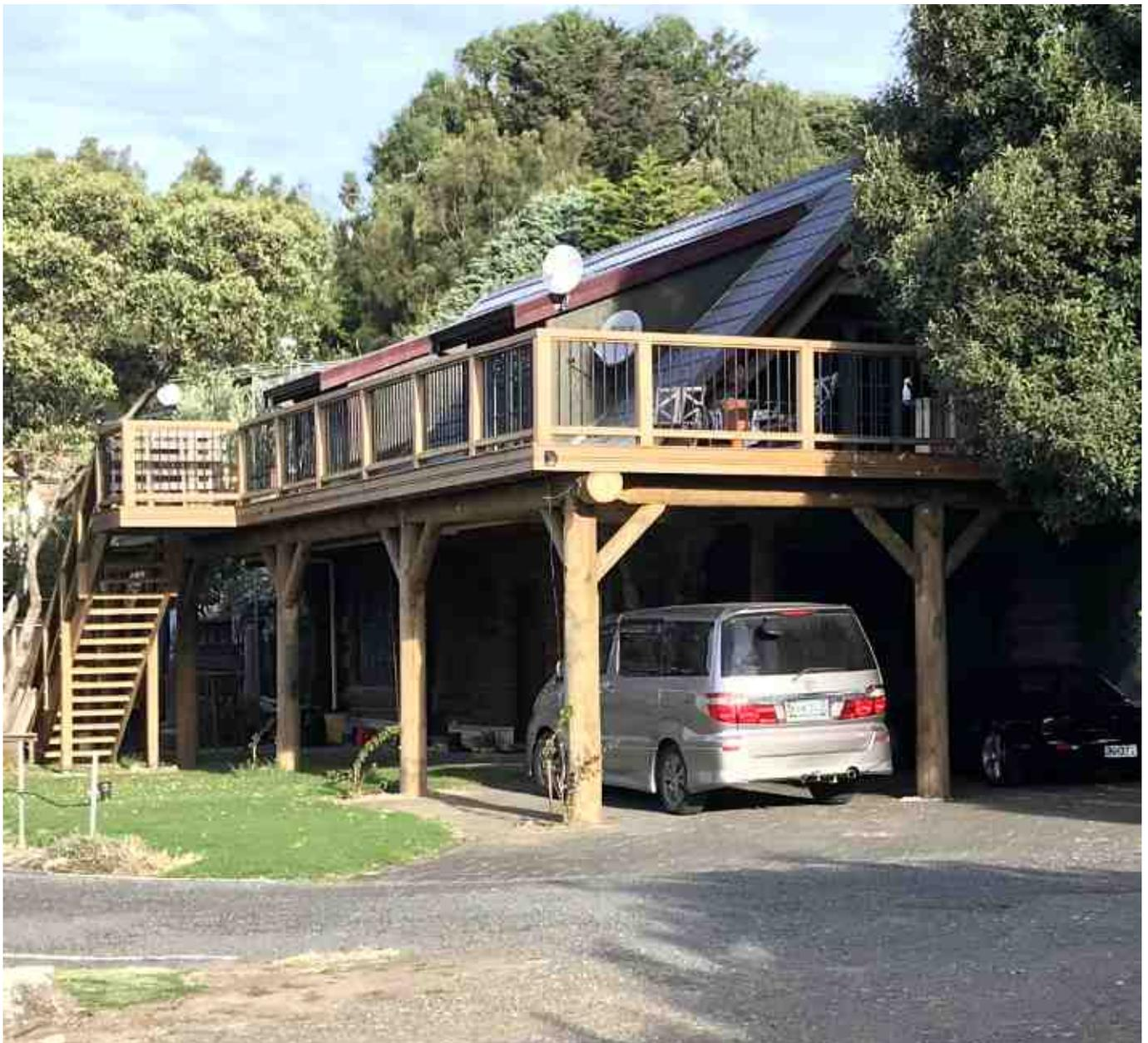
*Here is an overall view of the decks surrounding Cappamore. The extended deck acts as a carport and provides tons of elevated outdoor space off the upstairs french doors. The new stairway is not only beautiful, but is a safety feature as an emergency exit from the upper level.*
