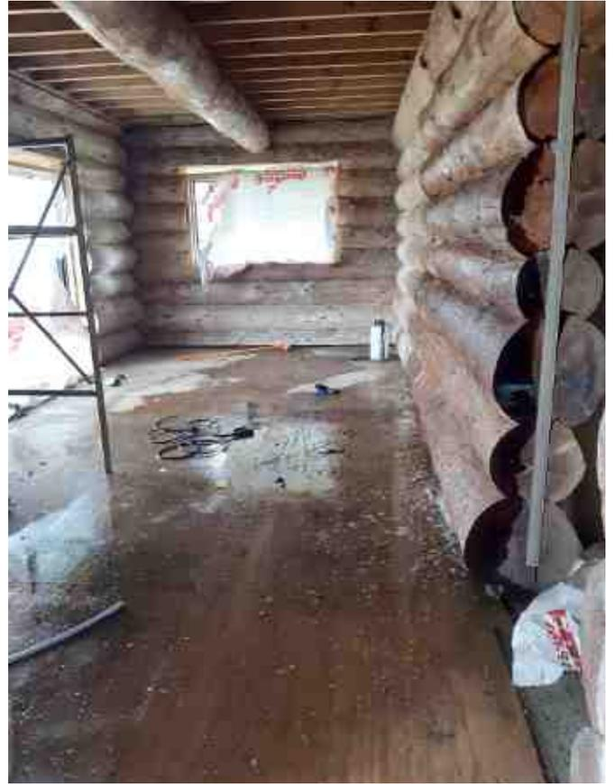
*Top left and right: Wet floors after waterblasting the inside logs to prepare them for oiling.*
