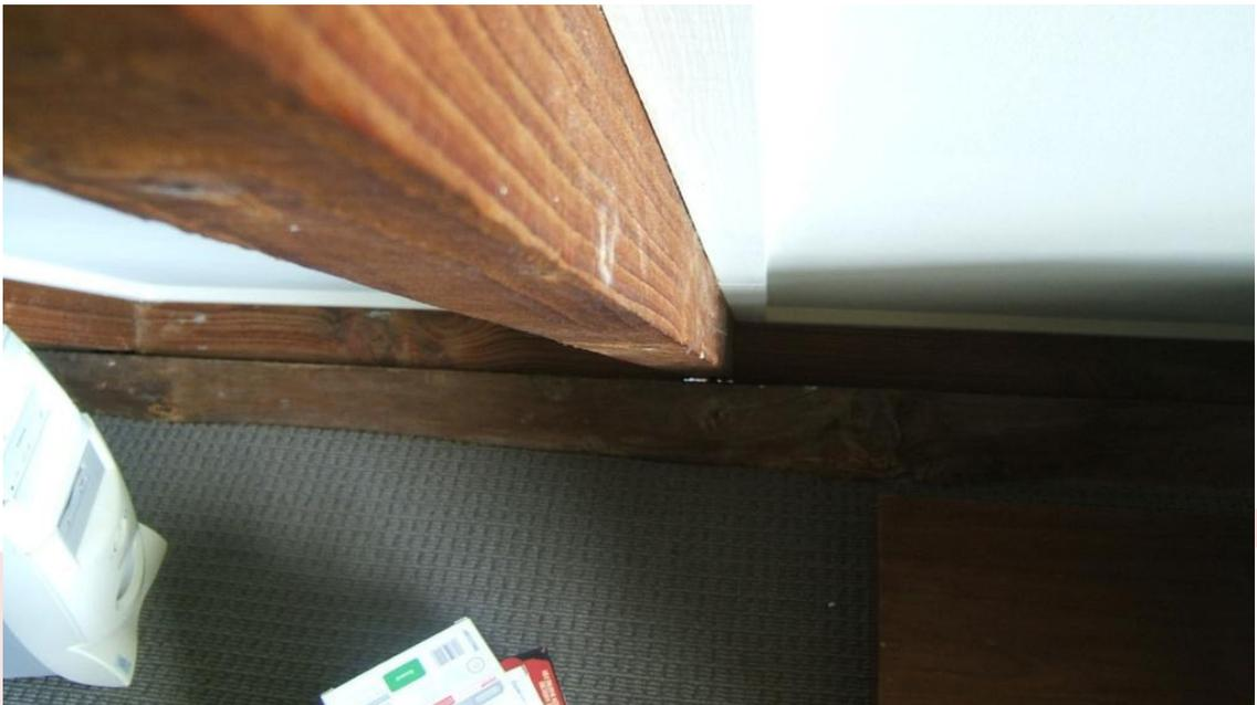
*Rafter to Log Wall Fixing Separation (note daylight between rafter & log)*
